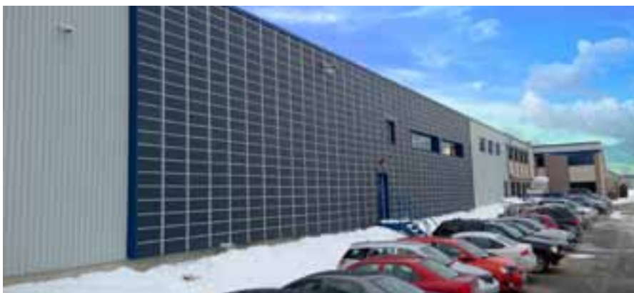
The facility in Magog, Canada, invested in what is known as a solar wall. The new technology resulted in a reduction in gas consumption of nearly 20%.
